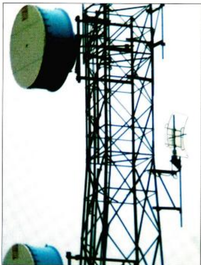
The ATTC DOCR receive antenna had a direct line-of-sight view of the primary station 42 miles away. The antenna was mounted on a rotor to investigate the effects of antenna orientation and coupling in the DOCR antenna system.
